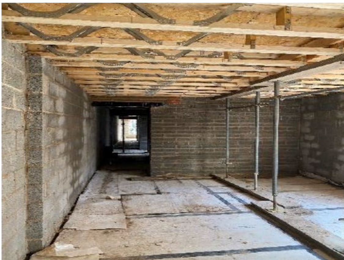
First floor rear flat bedroom, looking back towards flat entrance door
