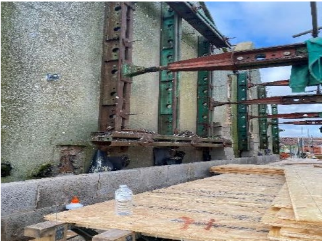
Third floor blockwork progressing
